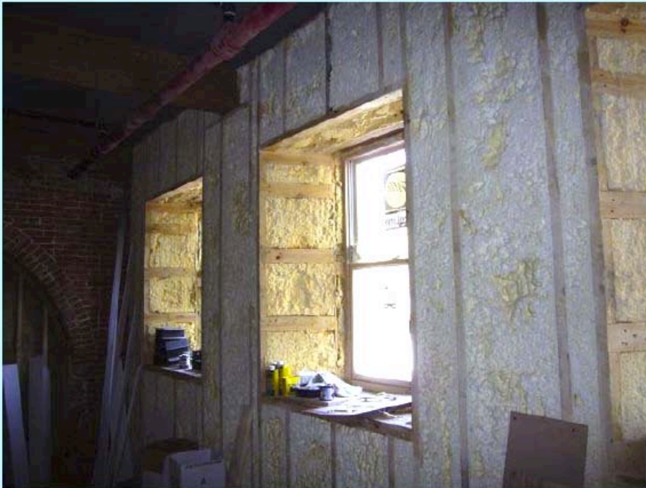
Interior spray foam of an historic bearing wall brick building
