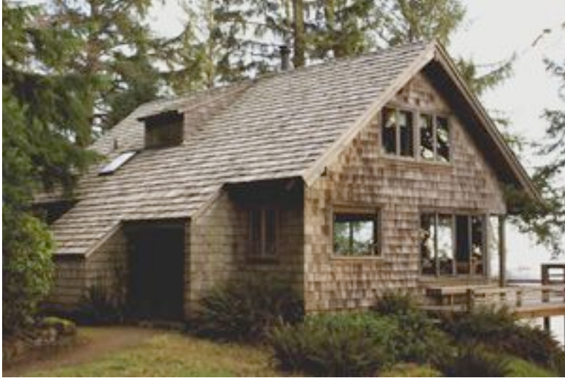
Left: Woodshed and entry porch are on the north, out of the coastal winds.
